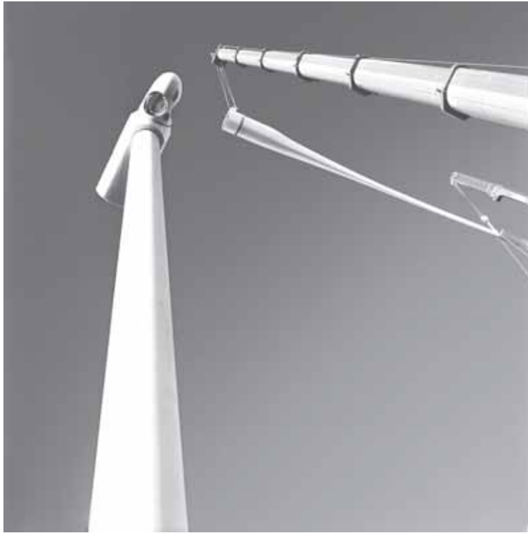
Figure 10 Installation of wind turbine blade.
