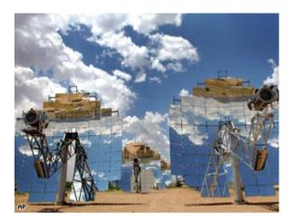
CSP provider Stirling's dish assemblies soak up the sun at an air force base in New Mexico.
