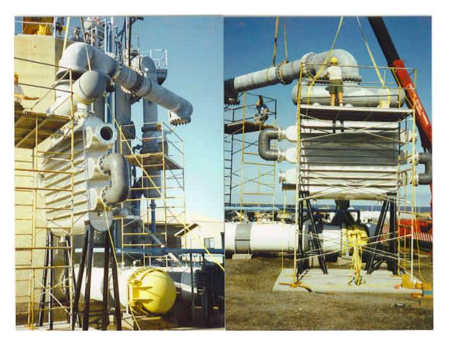
Aluminum plate-fin heat exchanger with extruded water passages and bonded with navy epoxy as a surface condenser in the open-cycle test facility
